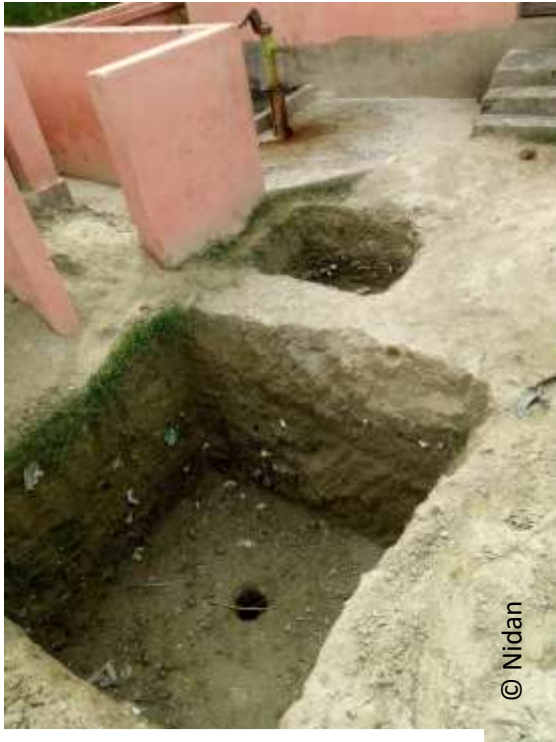
Construction of soak pit in Barbatta in 2019
